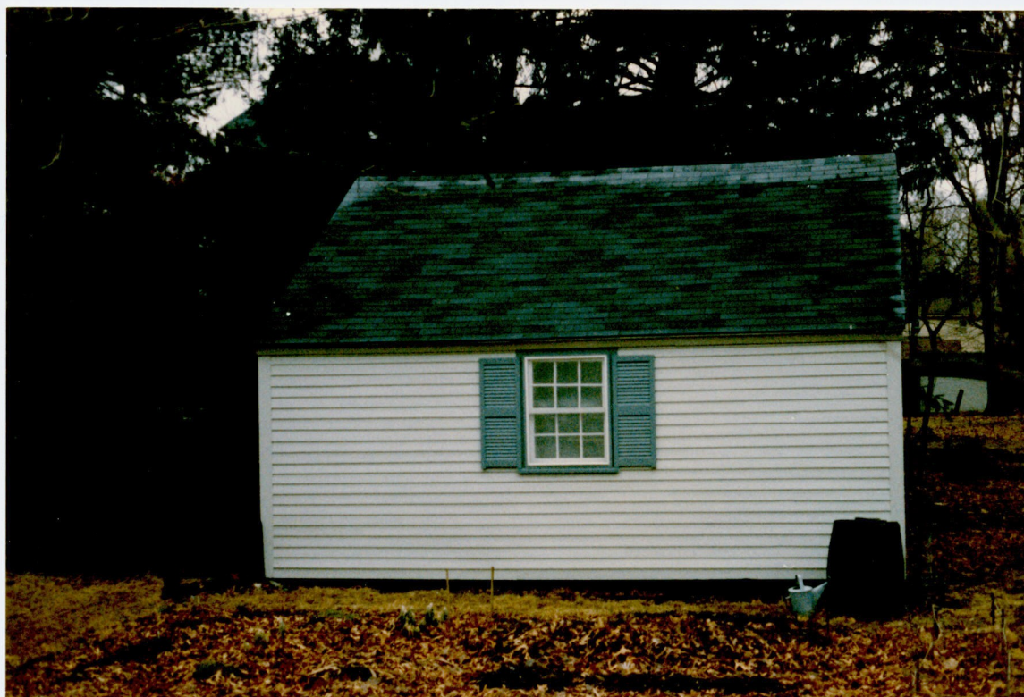
W-6 PHOTO OF GARAGE, RIGHT SIDE VIEW (FROM CANTON AVE)
