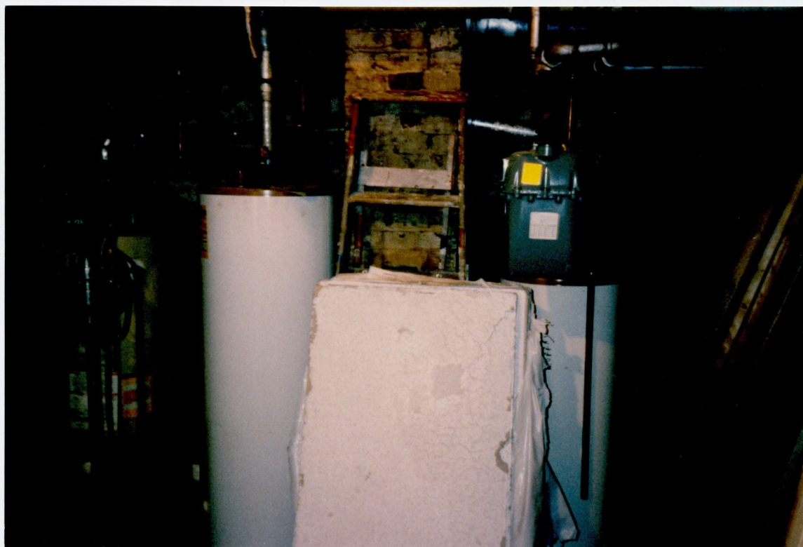
A-17 PHOTO OF THE BACK ROOM. IN THE CENTER OF THE PHOTO ARE THE BROKEN CEILING TILES FROM THE FRONT ROOM. TO THE RIGHT IS SOME MORE OF THE WOOD FROM THE BOXES THAT BRIAN OLEARY BUILT FOR THE CSM HELICOPTER LIFT, AND TRANSPORTED BACK TO THE OFFICE ON THE 19th OF OCTOBER BY NURDAN, DAVE, RICH AND MYSELF. TO THE LEFT OF THE PHOTO IS TWO PHOTO LAMPS FOR UTILITY LIGHTING ON CERTAIN JOBS. THE THREE ROUND OBJECTS IN THE BACKGROUND ARE THE WATER HEATERS FOR THE UPSTAIR TENNANTS. THE LADDER BEHIND THE CEILING TILES BELONGS TO TOM PETERS THE LANDLORD.
