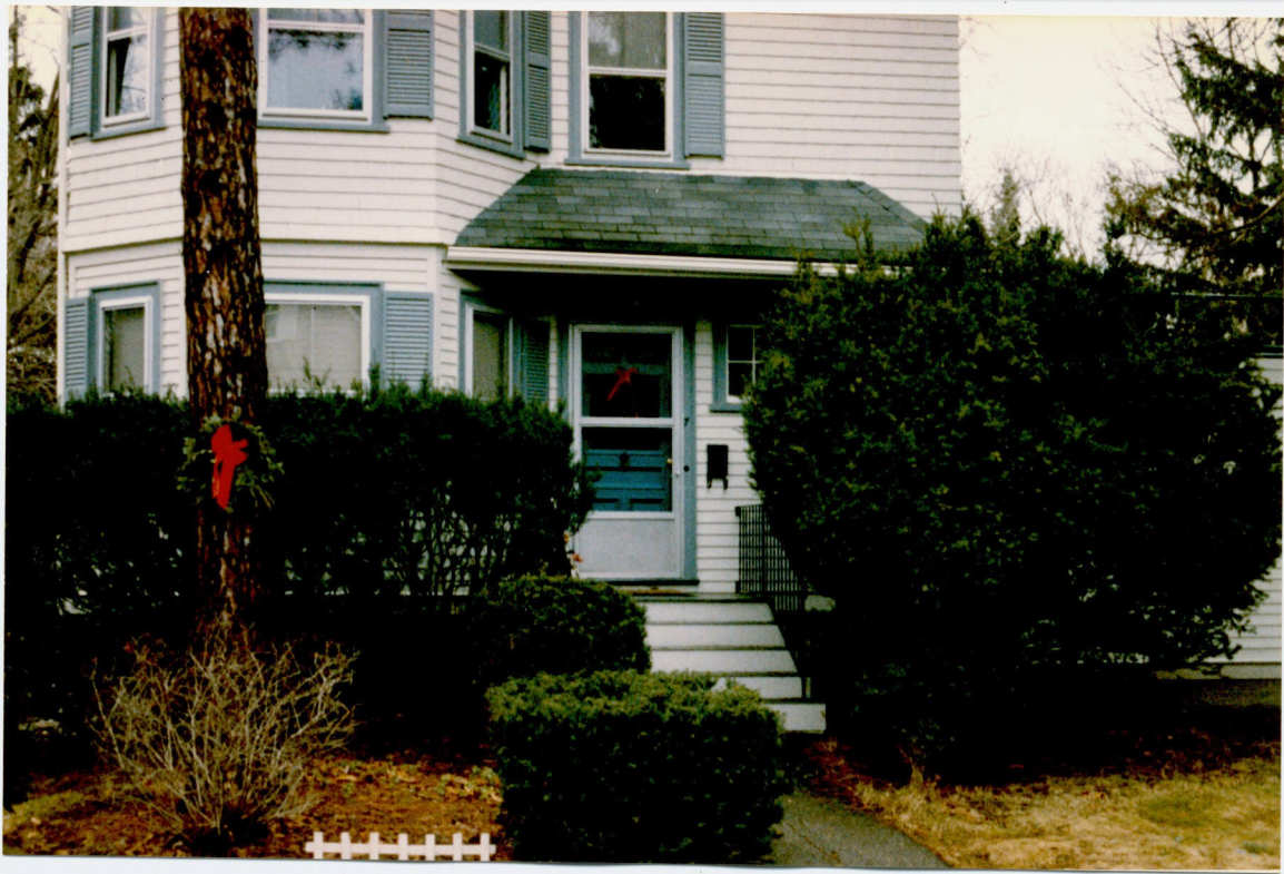
W-3 PHOTO OF 7 WHITELAWN AVE, FRONT VIEW
