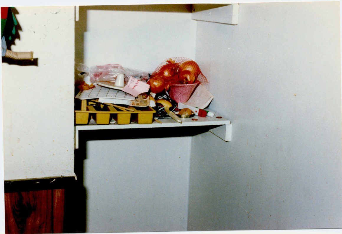
C-20 PHOTO OF BOTOM STORAGE SHELF, KITCHEN, WITH ITEMS REMOVED.
